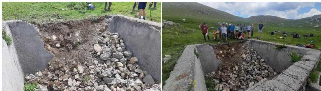
Picture 1 and 2. Water well made safe for bears and wildlife
